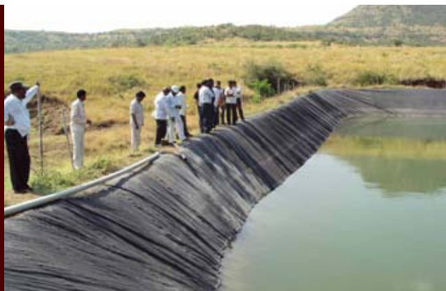
Water tank with polythene sheet in the bottom
