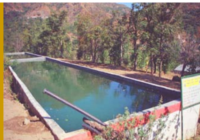
Common Tank with 4,40,000 litre capacity under NREGS irrigating agriculture with user charges – Nauni Panchayat, Solan Block
